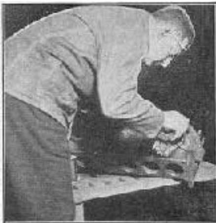
Fig. 4-Cleaning the vee with a wire brush
